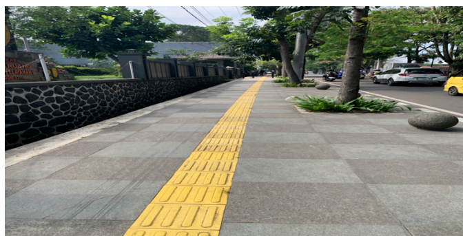
Figure 1. Sidewalk on Bhayangkara Road with Guiding Block and Bollard
